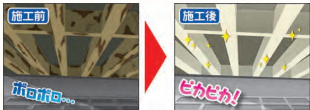
BA-3003 (橋桁塗替工事)
